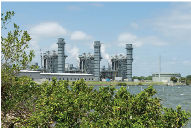
1,200MW plant in Florida
